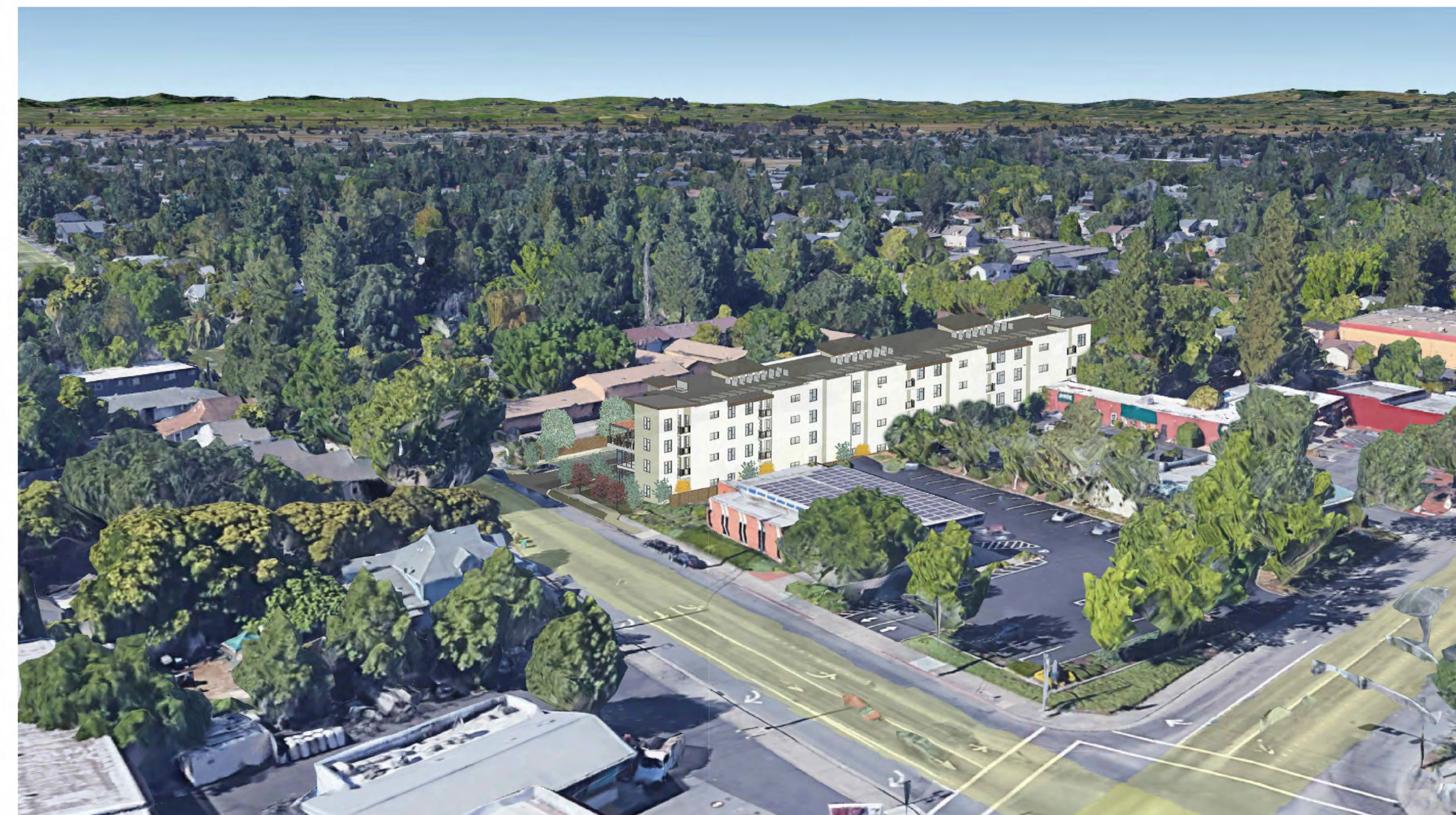
Aerial View from Northeast
